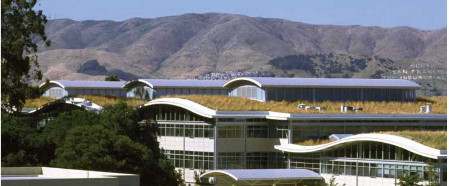
A green roof on the offices of YouTube in San Bruno, California.
