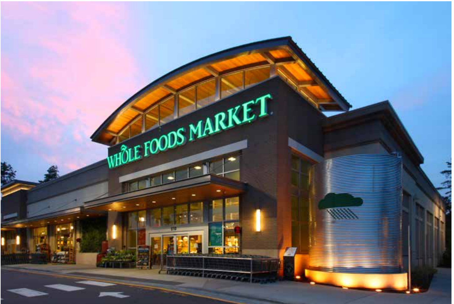
This cistern at a Whole Foods Market in Raleigh, NC, collects rainwater for interior restroom use.
