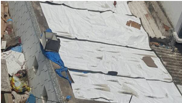
Pictures showing cool roof pilot installation and testing underway in Hyderabad, May 2017 (photo: ASCHIIIT-H)
