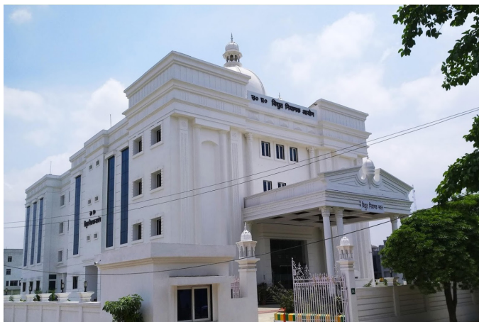
U.P. Electricity Regulatory Commission Building in Lucknow, ECBC Compliant and GRIHA 5 star rated
